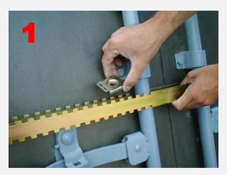
1.) Position NEW FORKSEAL between the central barriers of the container and insert the first joint the closest possible to the barrier...
